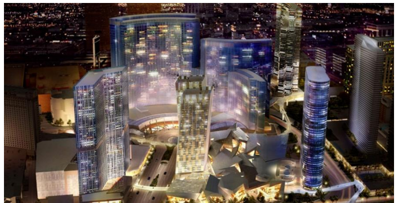
City Center – Las Vegas, NV Client: Beck Steel, Inc. – Design of more than 300 stairs and misc. structures for the Aria Resort & Casino and the Mandarin Oriental Hotel & Casino portions of the complex within a very tight delivery schedule.
